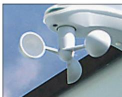
If there is a control system, the mechanical wind sensor should be checked periodically for damage from external causes and that it is functioning. Check that it turns in the wind. If it does not turn correctly, it must be checked by a STOBAG specialist supplier.
