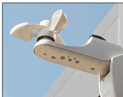
The installed mechanical and electrical wind sensors are maintenance-free. Please refer to the sensors' operating instructions accordingly. The mechanical wind sensor should be checked regularly to ensure that it is functioning properly (observe rotation behaviour in windy conditions).
